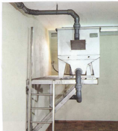
Separator with inlet at the top. The filtered water is discharged at the bottom.
